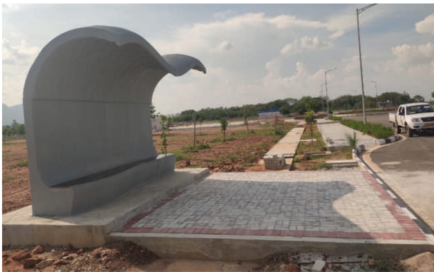
Bus stop build using 3D concrete printing technology
