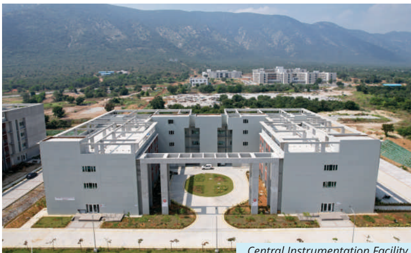
Central Instrumentation Facility
